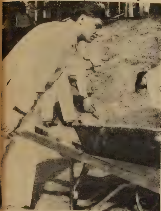
This Skuleman is working out his initiation at Bickford Park. First Year engineering students are working at this park to clear, grade, and dig the grounds. Shown here with the wheelbarrow is George Hildebrandt, I SPS. —VSP By Stan Klosevych
